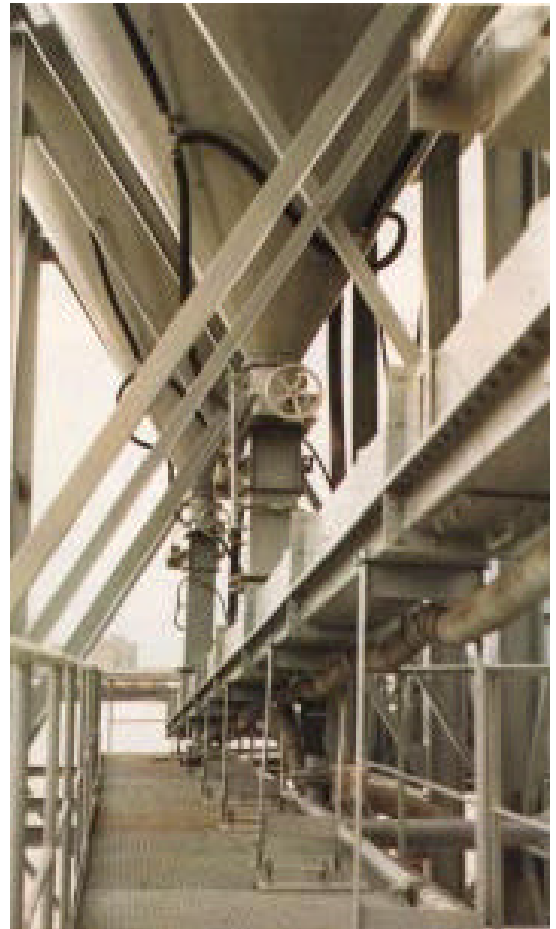
The above photo shows a typical Air-Slide with multiple inlet points
