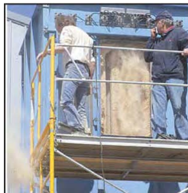
Bridged and packed baghouse.
